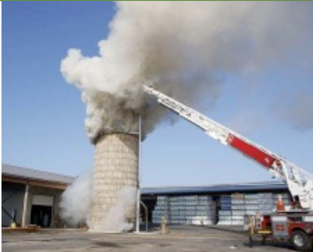
Fire in a silo containing wood chips; Lancaster, PA, December 2015; Lancaster Online.
