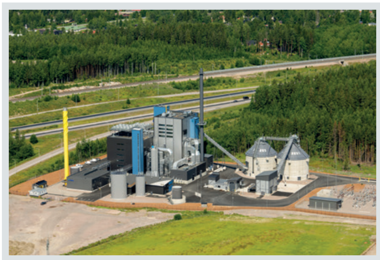
Figure 12 Aerial view of Järvenpää multifuel CHP plant
