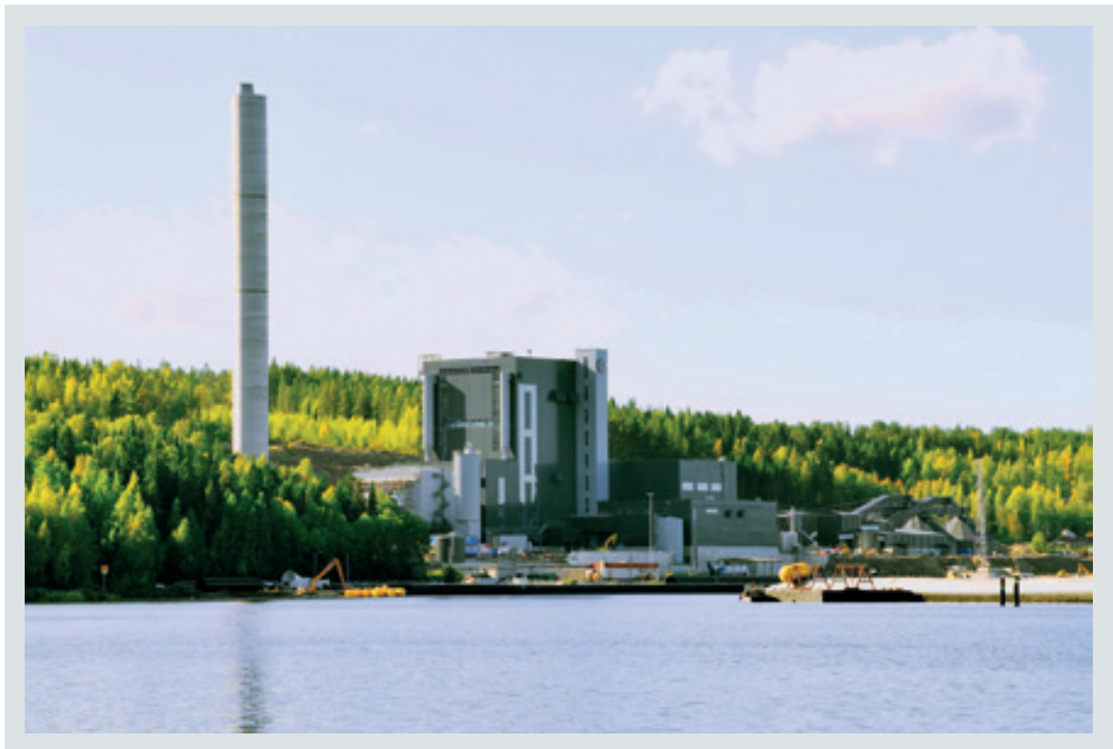
Figure 5 Keljonlahti CHP Plant in Jyväskylä
