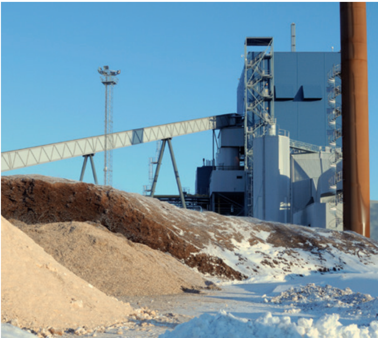
Typical Multifuel CHP Plant in Finland ( Sumitomo SHI FW Energia Oy )
