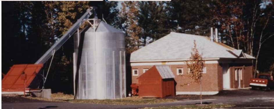
Lyndon Town School, Lyndon, Vermont System Size: 1.2 MMBH Manufacturer: Chiptec Wood Energy Systems This system uses an above-grade metal silo and separate boiler house (which includes garage space). Silo is loaded from a receiving bin (on far left) using an inclined auger.
