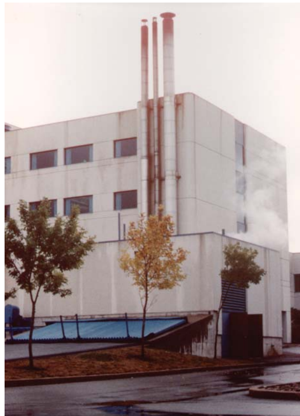
South Shore Regional Hospital, Bridgewater, Nova Scotia System Size: 4.0 MMBH Manufacturer: KMW Energy Systems Showing top-hinged hydraulically operated loading doors for below-grade bin adjacent to boiler room.
