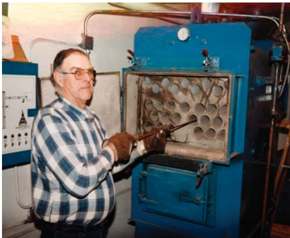
Boiler Tube Cleaning Manual boiler tube cleaning shown at Calais Elementary School, Calais, Vermont (.5 MMBH system by Messersmith Manufacturing).
